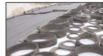
Figure 18: Use of gravel filled bags (left) and tires (right) to weigh down plastic covering
